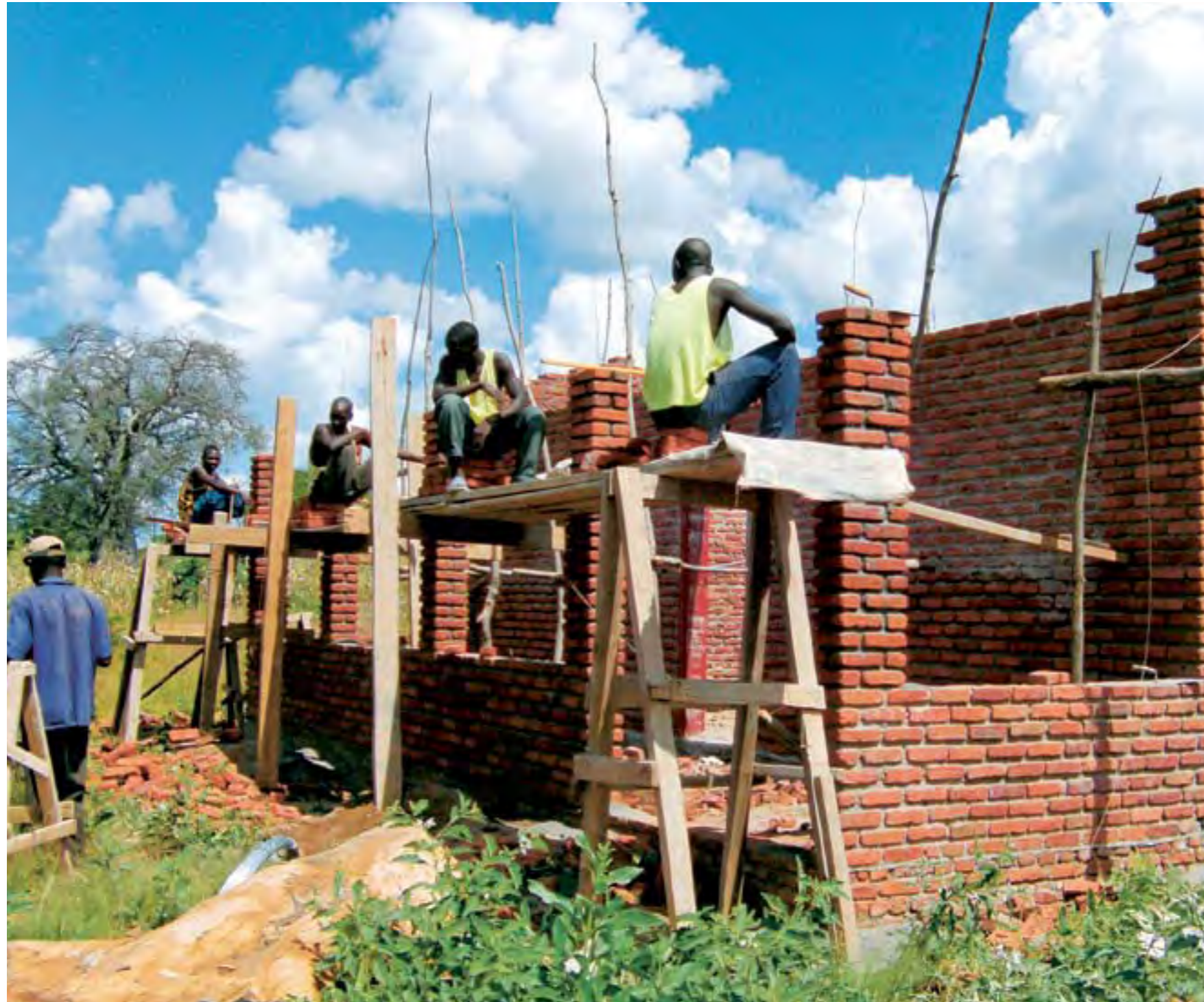
Construction of the Salima Secondary School Campus, Malawi
