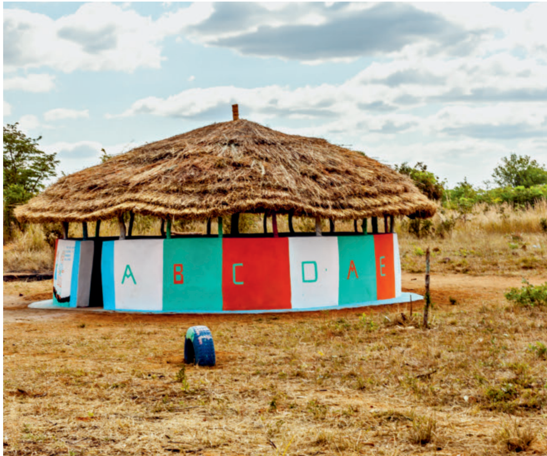
New early learning center built by a community in the Lundazi District, Eastern Province
